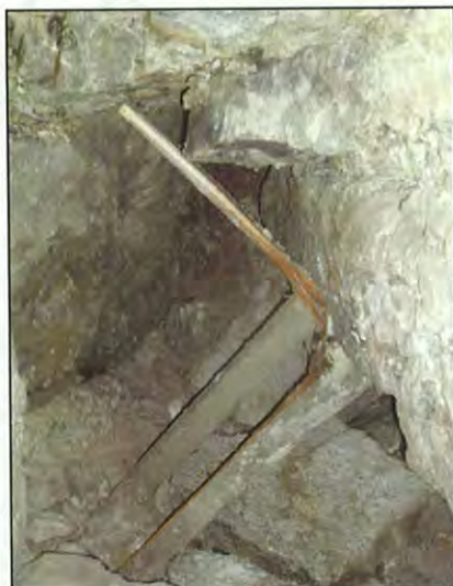
Wooden struts support the side wall
