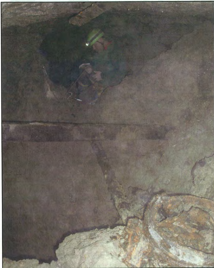
Kibble, Pipe and Beam
