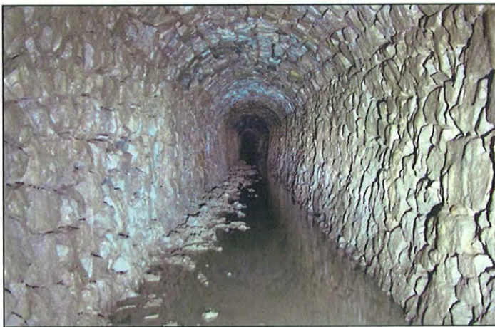
The ginged walls of the main adit
