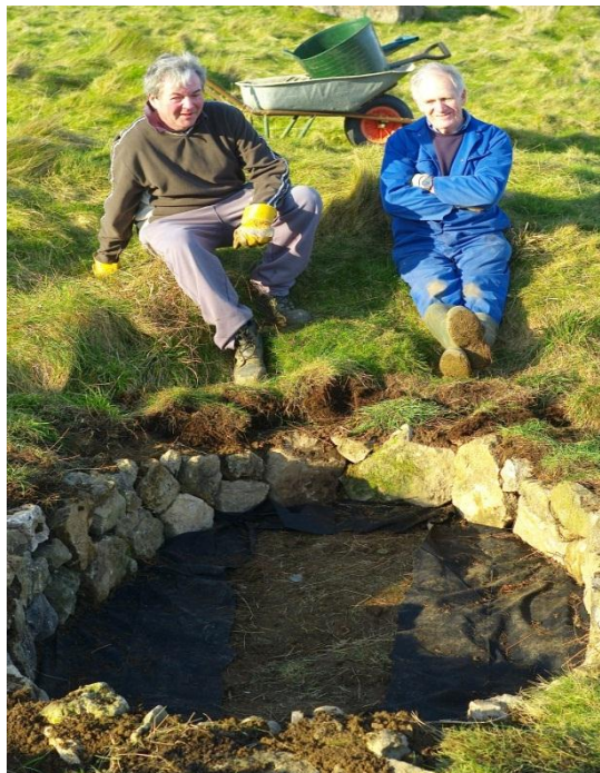
Steve and Brian taking a break from pit reconstruction work
