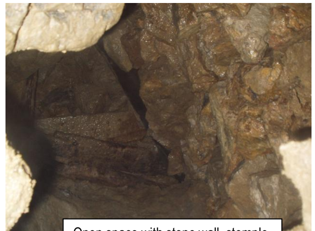
Open space with stone wall, stemple and wooden shuttering.
