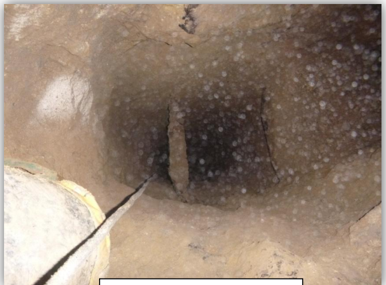
Looking down Graceland Shaft
